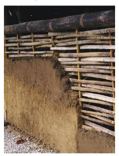
**Figure 1.** Sustainable building structure utilizing dried bamboo strips and adobe.
